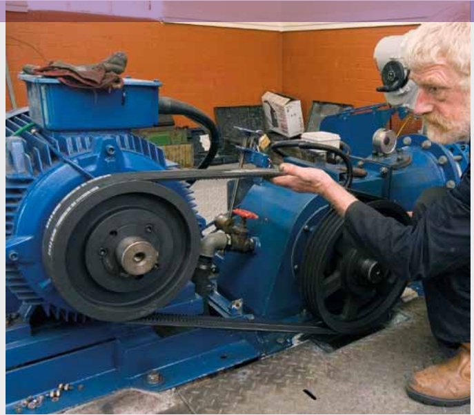
Hydroelectric turbine, Talybont Reservoir
