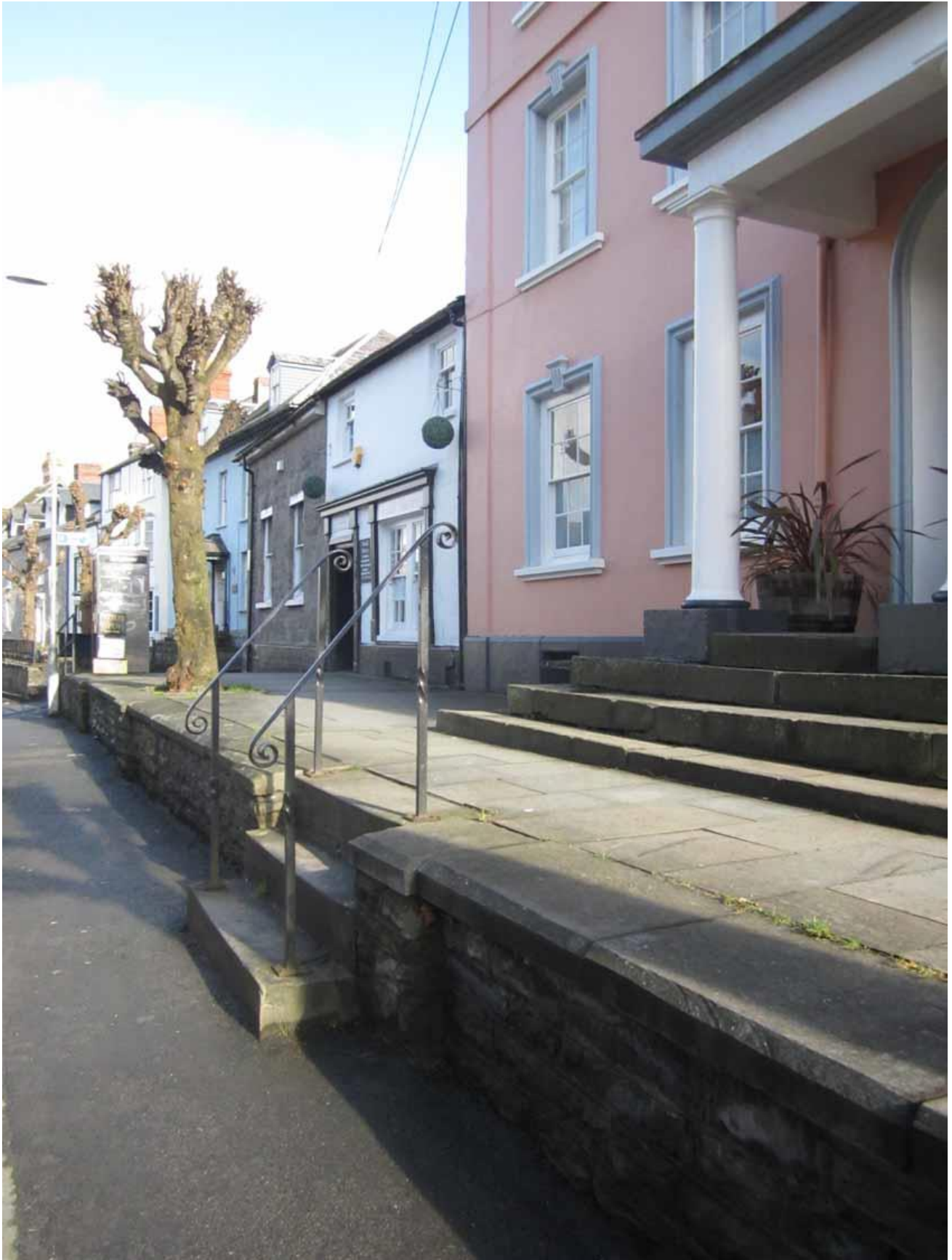
In Broad Street, the low retaining wall and natural stone paving on the raised pavement above are augmented by metal railings which help reinforce the steps between the two levels
