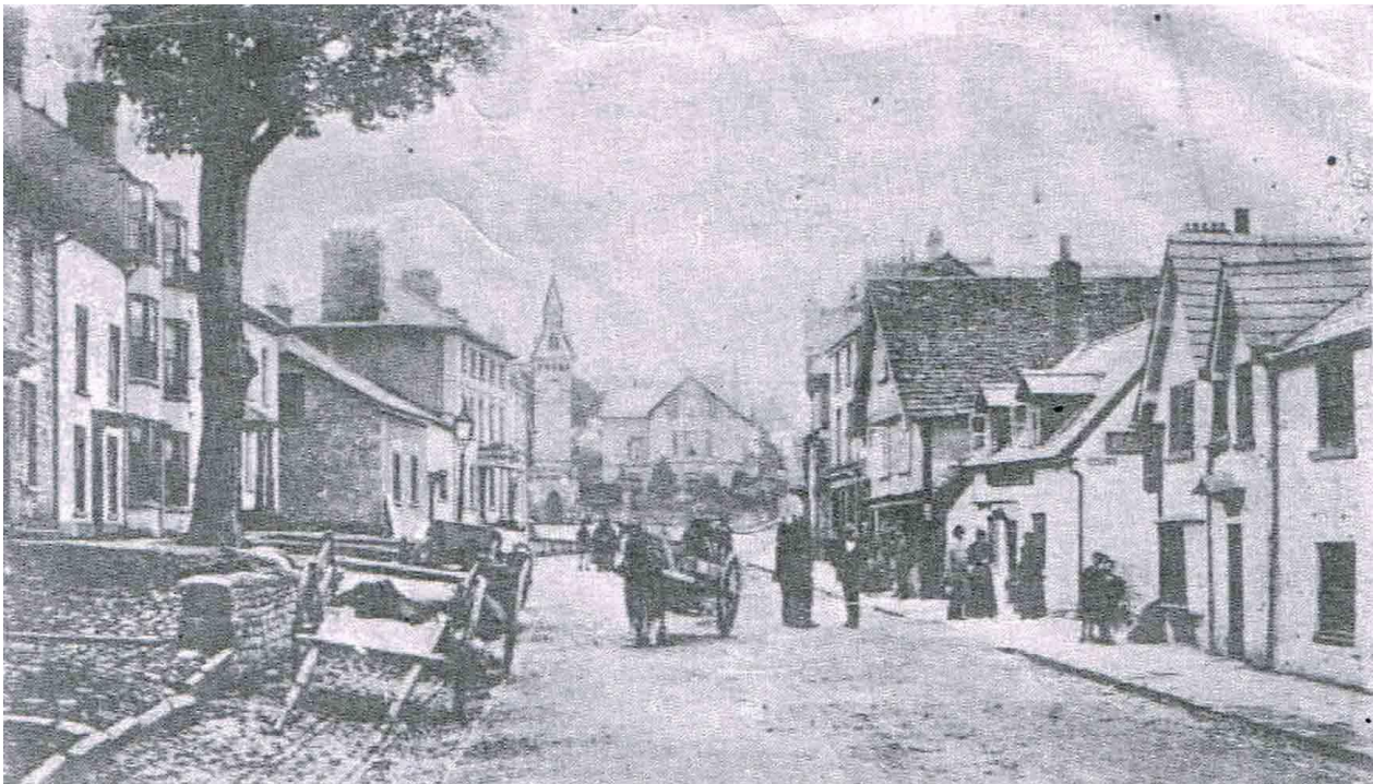
Broad Street 1905, looking south towards the Clock Tower
