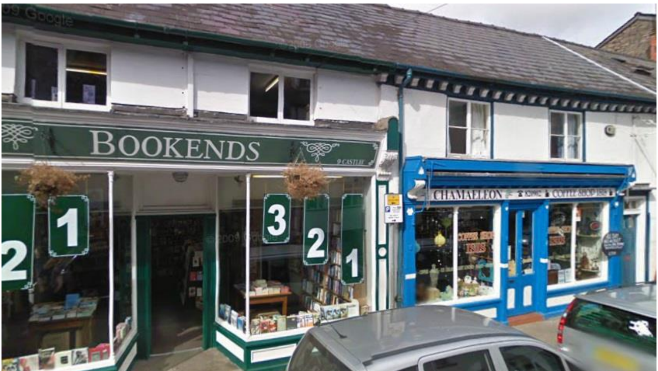
Traditional shop fronts in Castle Street
